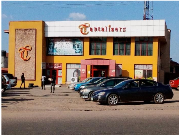
Plate 5; Exterior of Tantalizers
