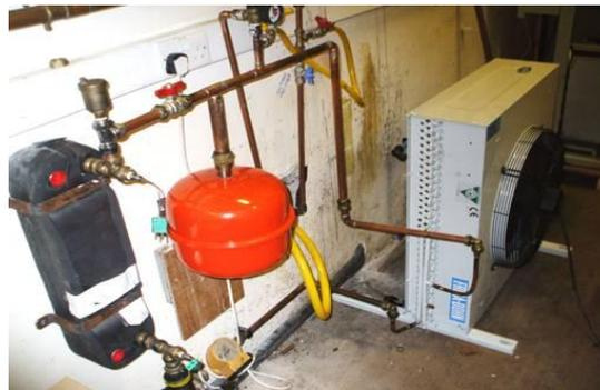
Figure 15. Shows the connections of the heat exchanger, water pump, heat rejection fan and expansion valve.
